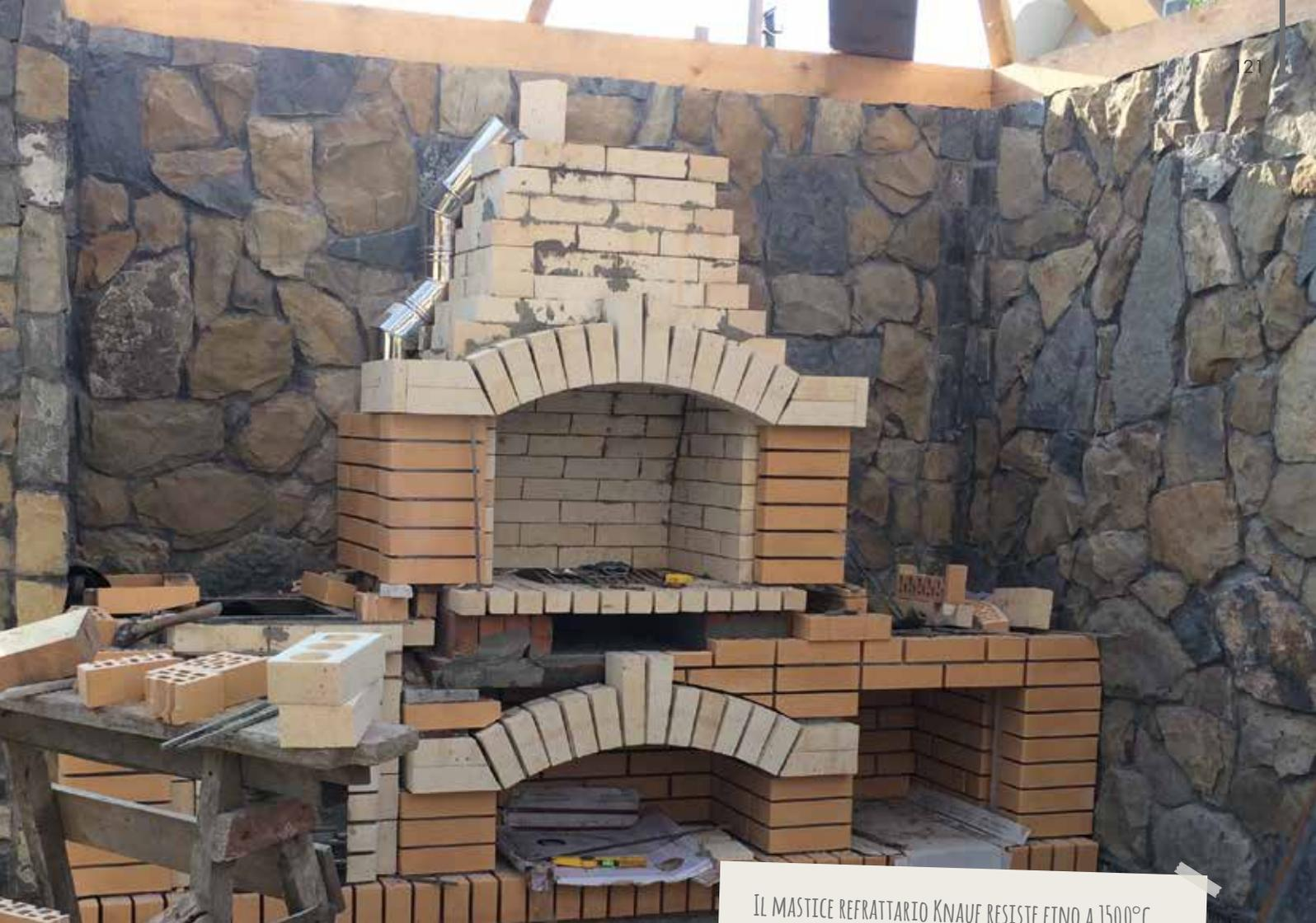
IL MASTICE REFRAATTARIO KNAUF RESISTE FINO A 1500°C
