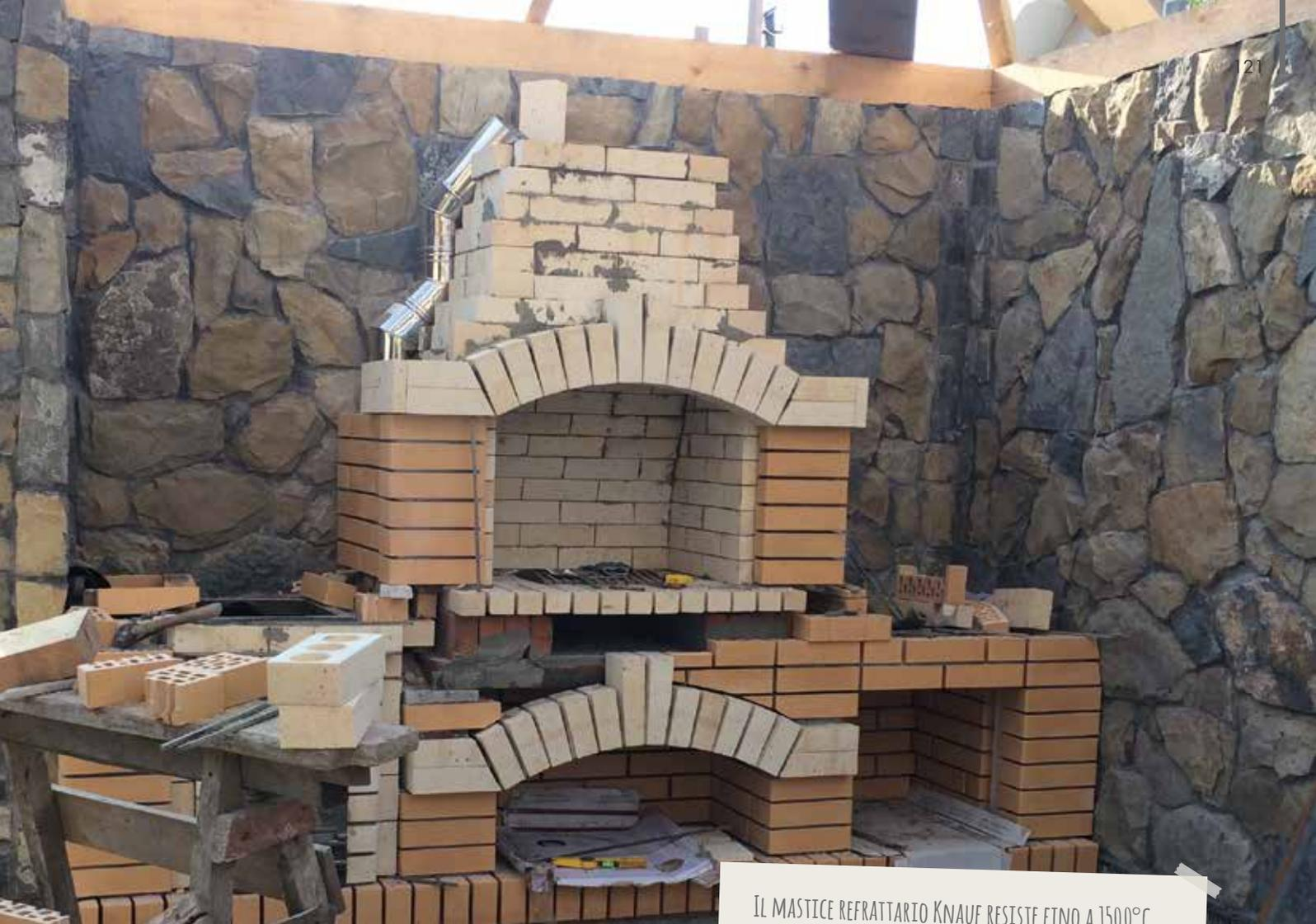
IL MASTICE REFRATTARIO KNAUF RESISTE FINO A 1500°C
